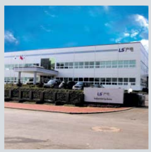
Dalian Plant (China)
